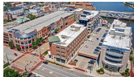
1st Street Development, St. Charles: 5 mixed-use buildings, including 16 affordable apartments.
