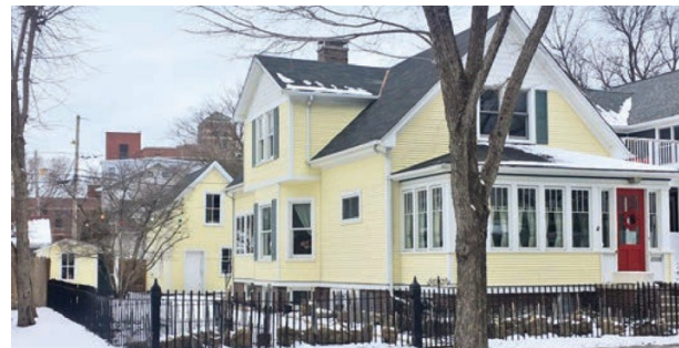
A coach house ADU , a type of ADU located above a rear garage, with design features that complement the single-family home.
